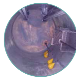
stations de relevage
